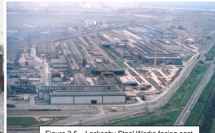
Figure 3.5 – Lackenby Steel Works facing east towards Redcar Steel Works in the 1980s
